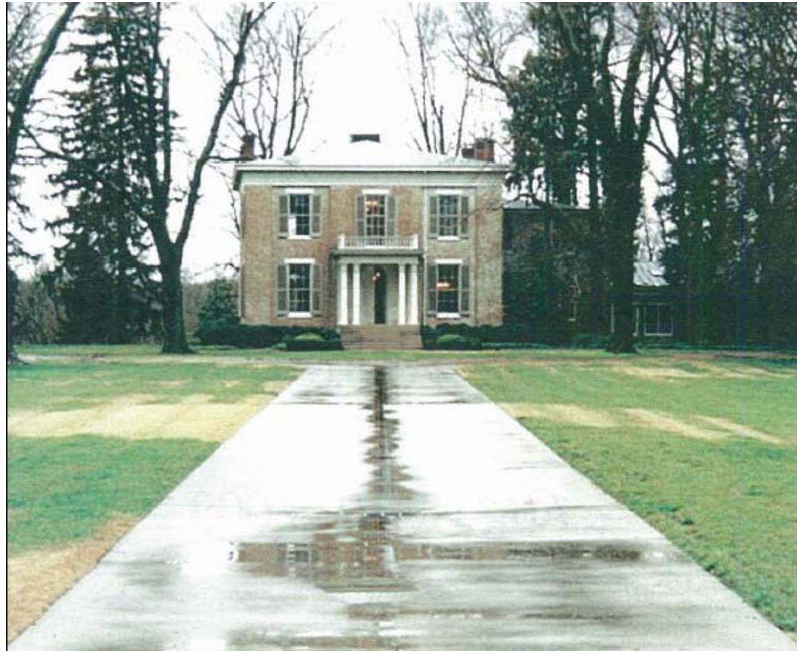
Rosewell Treatment Plan and Stabilization
