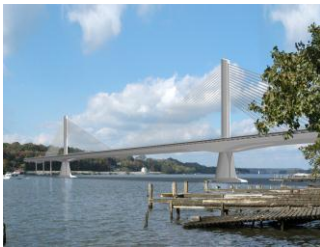
The East End Bridge has two towers in the median with cables giving it a sailboat appearance.
